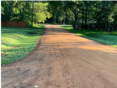
Albert St. reconstructed, waiting on cement treatment.
